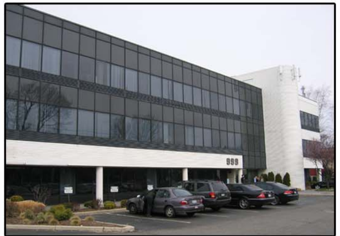
999 Walt Whitman Road Melville, New York 25,000 square foot office building
