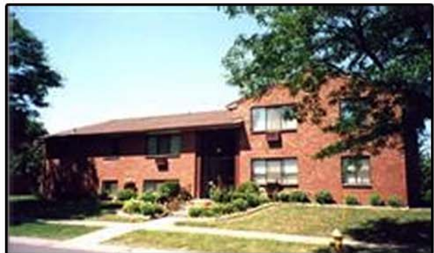
The Grecian Garden Apartment Complex Greece, New York 267 Unit Apartment Complex
