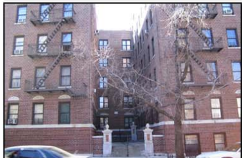
5 Apartment Buildings 217 Units Bronx, New York
